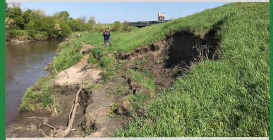
Photo, above: Erosion near a USACE operated levee along Salt Creek within the Salt Creek tiger beetle's range.
