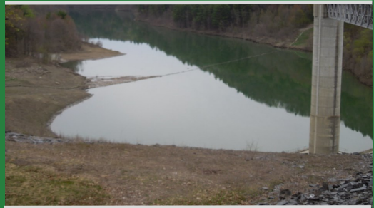
Photo, left: An image of the dam at North Hartland Lake.
